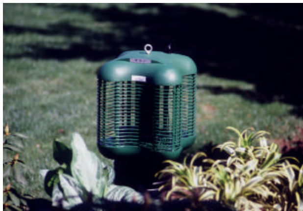
Figure 2 In-ground pedestal
